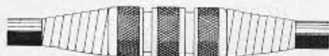
WIND PLASTIC ELECTRICAL TAPE AROUND CABLE IMMEDIATELY BEHIND CONNECTORS TO PROVIDE A SMOOTH CONTOUR BETWEEN CABLE AND CONNECTORS.
